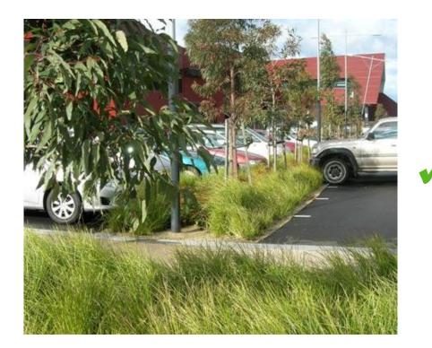
Figure 27 – Bio-retention system and swales
