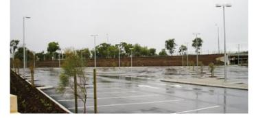
Figure 14 - Car park lighting that minimises spill light
