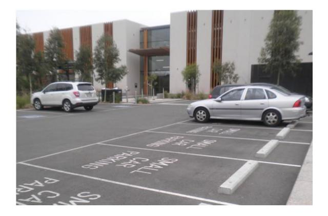
Figure 19 – Perpendicular small car parking bays
